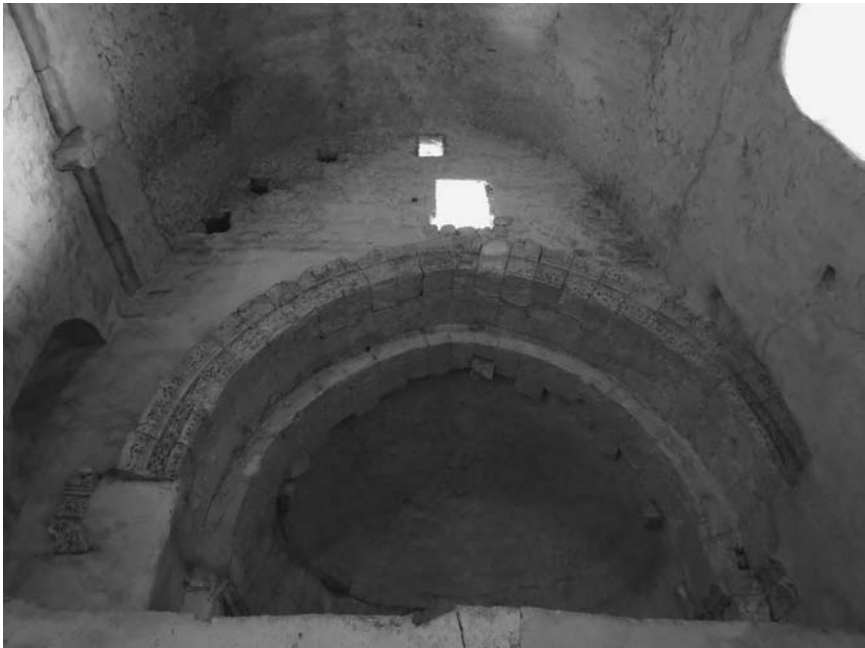
Fig. 2.2.11 Apse archivolt of the church of the Monastery of Mar Abraham of Kashkar
